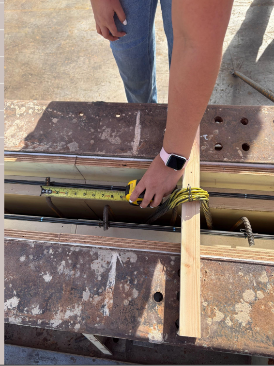
Figure 17: Verification of 7 in. stirrups
